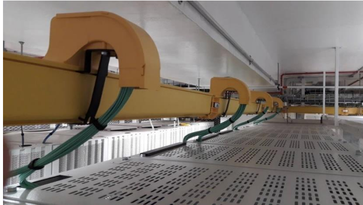
Figure 1.6: Fiber cables organized using Velcro
